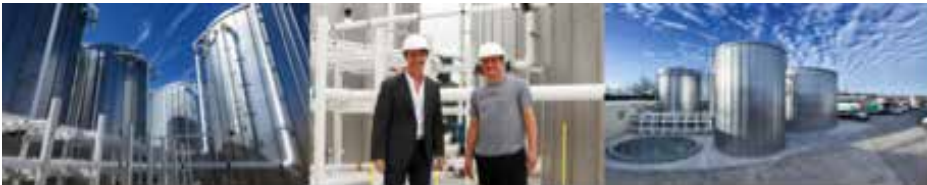
DPS's new wastewater treatment facility with Baswood founders Edward Norton and Woody Harrelson.
